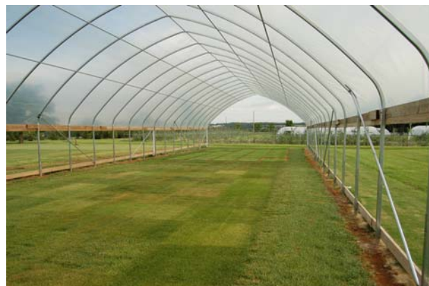
Figure 1. Fixed-roof rainout structure at Fayetteville AR
